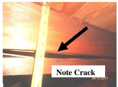
The roof rafters and/or roof framing of many older homes would most likely not meet current building codes and snow loads on these roofs can result in cracking of the roof rafters as seen in the picture to the left and/or loose connections for the roof rafters and/or roof framing members that can be seen in the picture to the right
