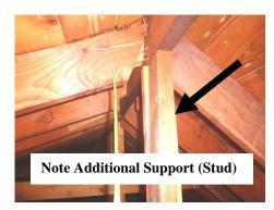
Some homeowners try to install vertical columns (studs) to provide additional support to the roof surface as seen in the picture to the left. This can lead to other concerns as this may shift the load (weight) from the roof to other areas that are not designed for the load such as cracking of the walls and/or ceilings as seen in the picture to the right.
